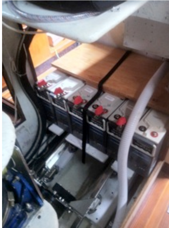
New Motor Mounts, Battery Platform, and Unfinished Wire Platform
