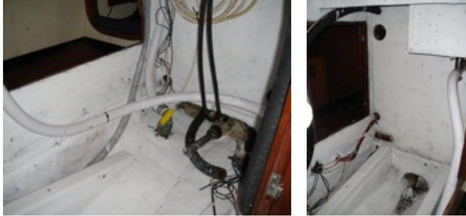
Motor Compartment - After a few Coats of Paint
