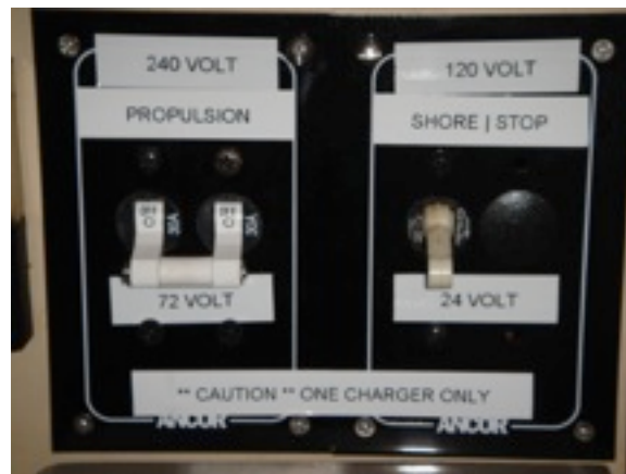
Charger Circuit Breakers - New Panel will Physically Ensure Single Selection
